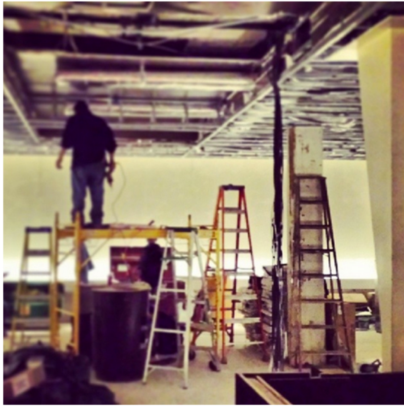
[The build-out begins.]
